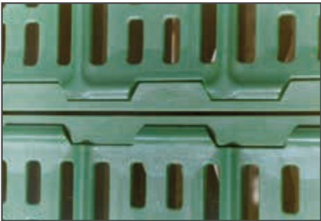
expansion gap with edge strip
